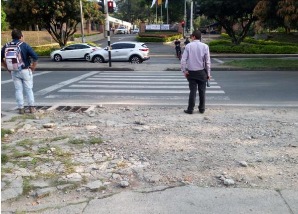
A photograph of a crosswalk at an intersection. The curb on the left side is severely damaged, with large sections of concrete missing, exposing the underlying gravel and soil. Two people are standing on the sidewalk, looking towards the crosswalk. A white car is visible in the background, and there are trees and buildings in the distance. |
