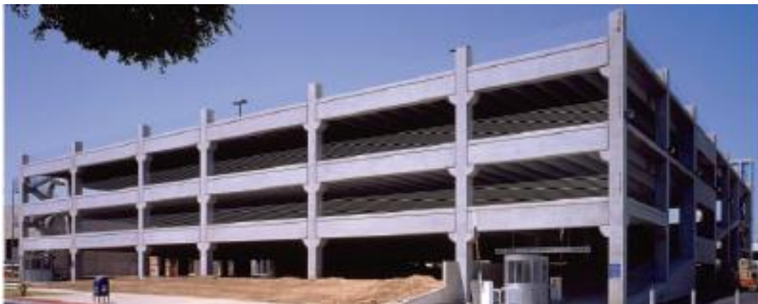
Figura 7. Wiltern parking structure, Los Angeles California (Extraído de https://www.dywidag-systems.com/ )
