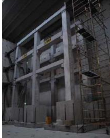
Figura 6. Ensayo de pórticos a escala real (NASCIMBENE, BRUNESI, BOLOGNINI and BELLOTTI. Experimental investigation of the cyclic response of reinforced precast concrete framed structures. PCI Journal, March–April 2015)
