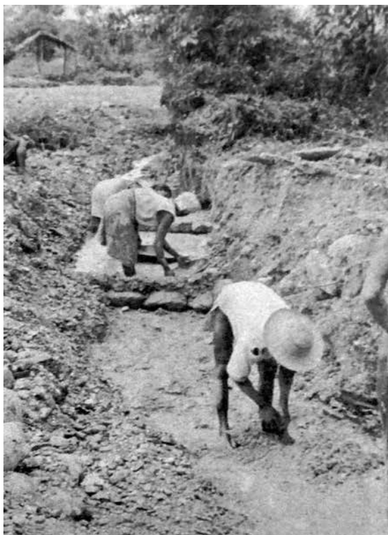
Figura 23. «The cleanup. Within the sluice the workers construct a small pond of water, in which the fine gold-bearing sand and gravel is washed with the batea» [«En la acequia los trabajadores construyen lavan las gravas con la batea»].
