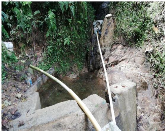
**Figura 18. Ingreso Bocatoma**
