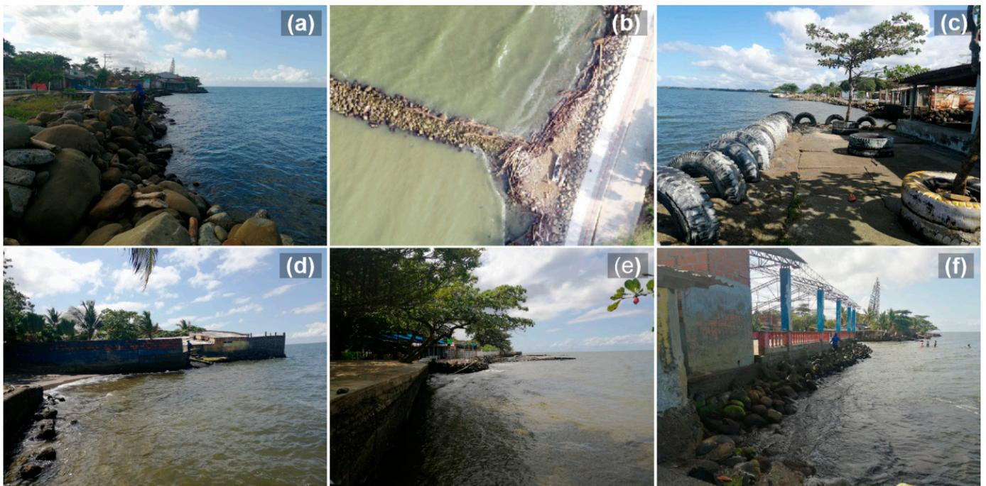
**Figure A2.** Types of artificial coastal protection structures associated with Table A1: (a) Rock revetment (structure 2); (b) Rocky groin (structure 4); (c) Seawall + Tires (structure 12); (d) Pentapod groin (structure 31); (e) Retaining wall (structure 20); (f) Rock + pentapod revetment (structure 13).
