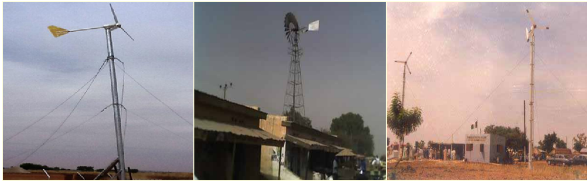
Figure 8. Wind turbines in some parts of Nigeria (from left to right): in Danjawa, in Kadawa and in Sayya, Gidan Gada [55,56].
