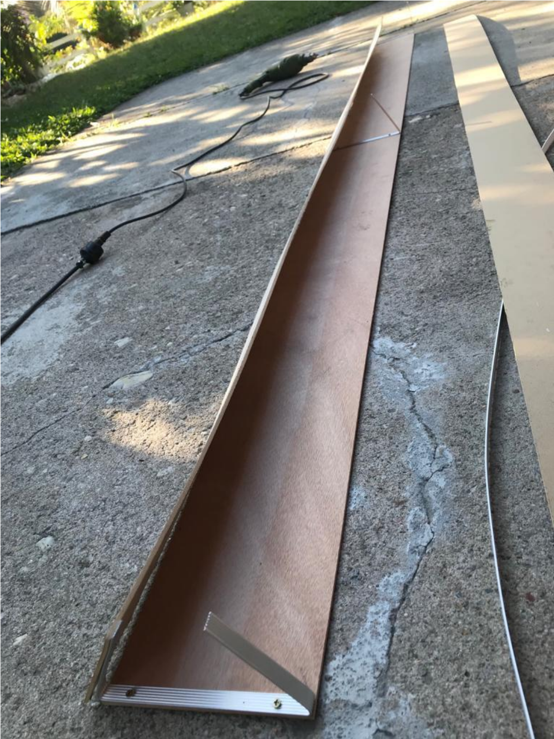
Fig. 41 Assembly of structure for the baffle. (Taken from own source).
