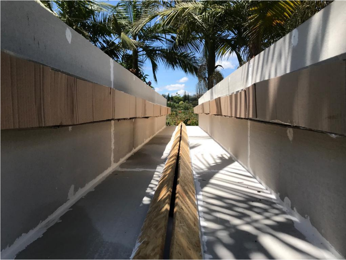
Fig. 50 Continuous balcony configuration with sound absorbing material on all sides. (Taken from own source).
