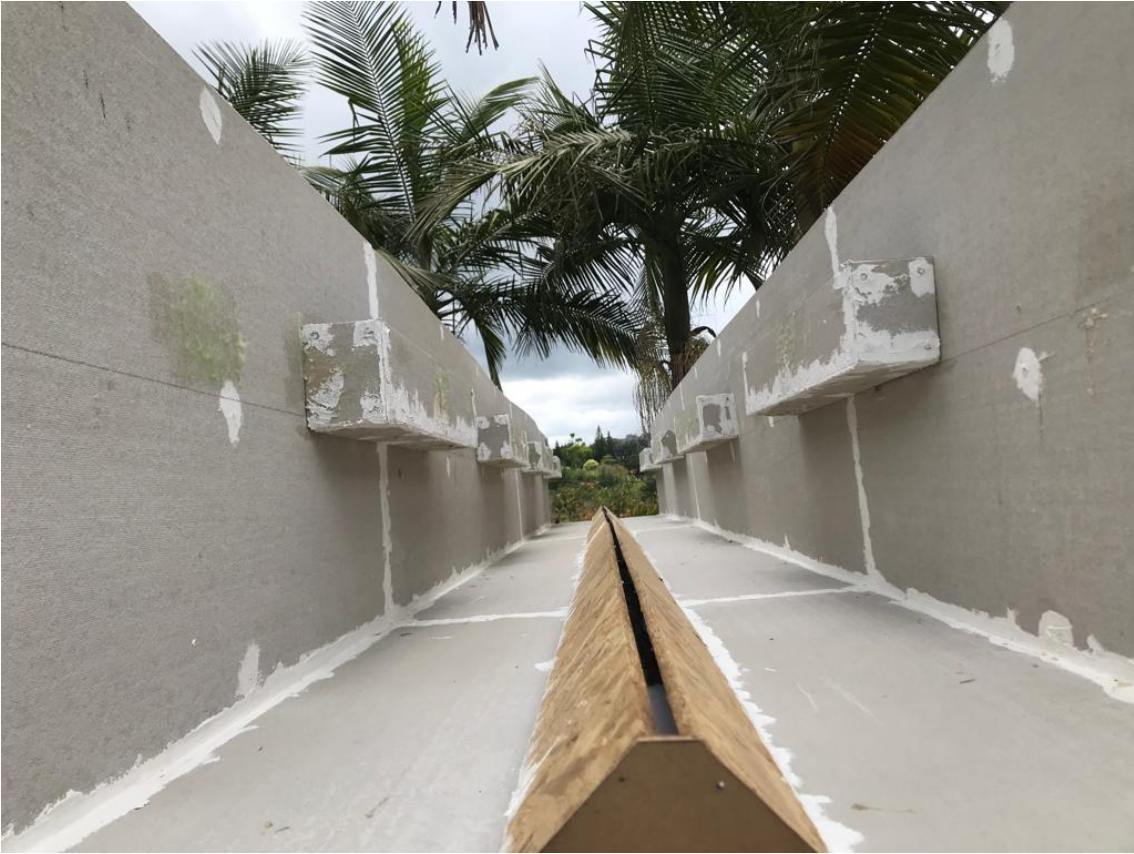
Fig. 48 Interspersed balconies. (Taken from own source).
