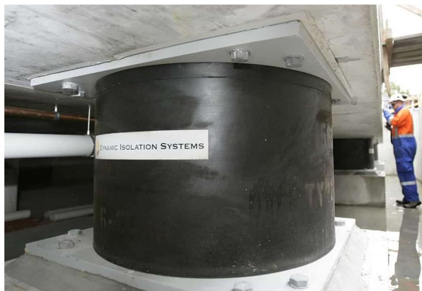
*Figura 4. Aislador elástico. (Recuperado de <https://civildigital.com/base-isolation-system-outline-on-principles-types-advantages-applications/base-isolation-for-a-building/>)*
